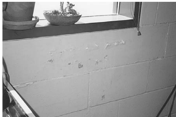
Figure 9-57 Vapor permeance of coatings affects moisture movement through walls and can inhibit evaporation or the wall's ability to "breathe."
